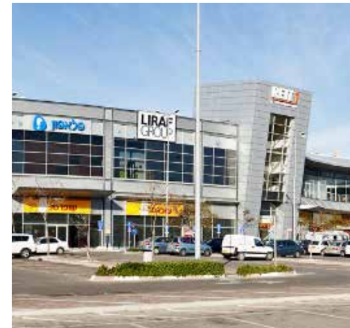
Power Center, Hadera
