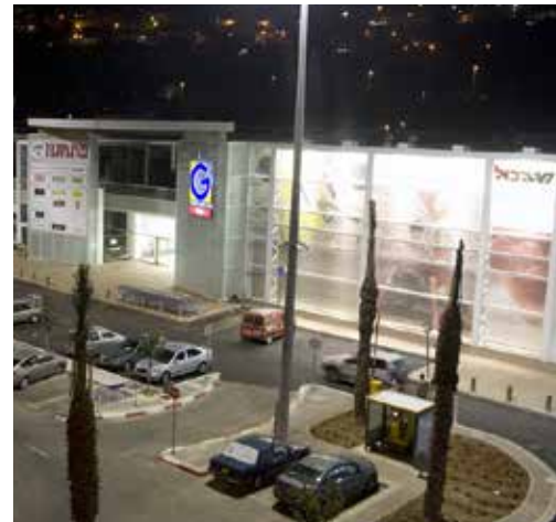
Power Center, Yoq'neam
